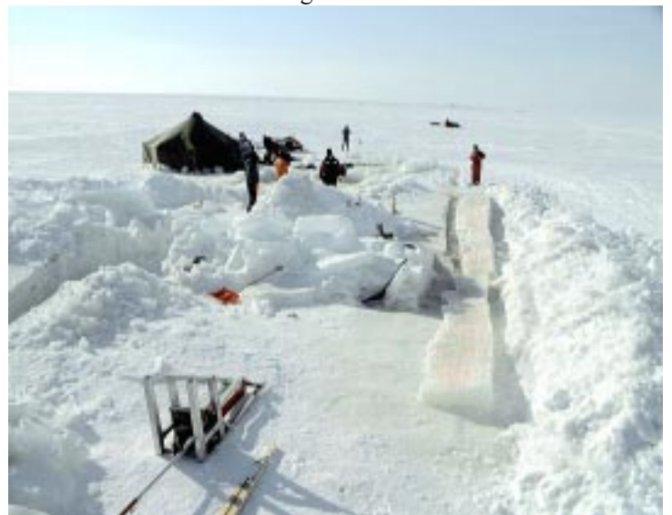
Figure 2. The consolidated layer cross-section is being built on the ice. Behind, the divers get ready.
