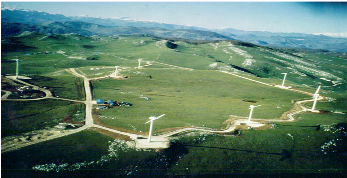
Fig. 1 - Top view of the Acqua Spruzza test site
